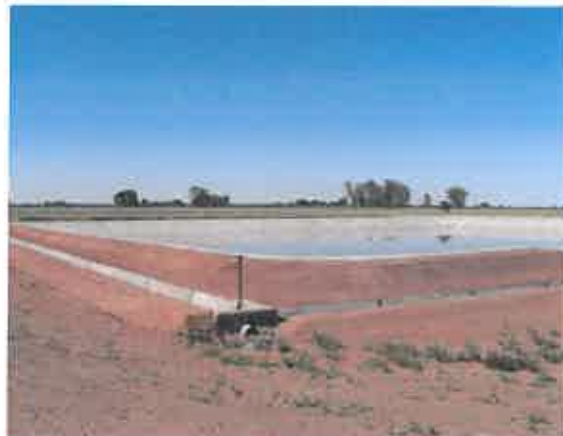
Ilima projects support: Completed reservoir at Vaalharts
