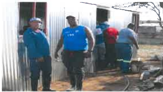
Pictures of the construction of the shack
