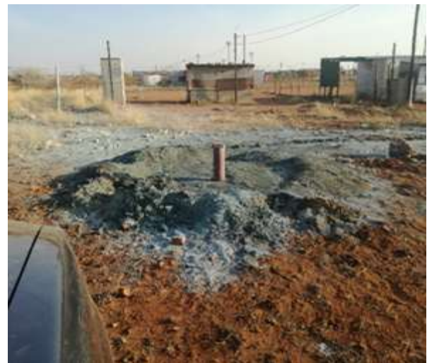
Drilling of the boreholes
