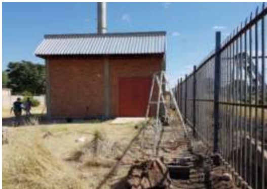
The incinerator at the laboratory
